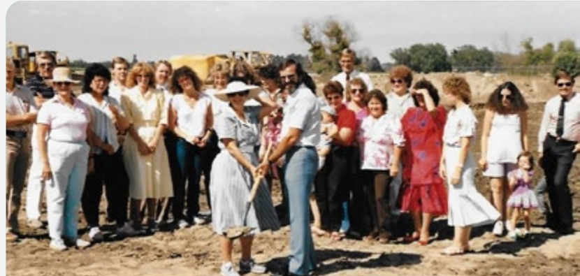
SJVC campus groundbreaking
